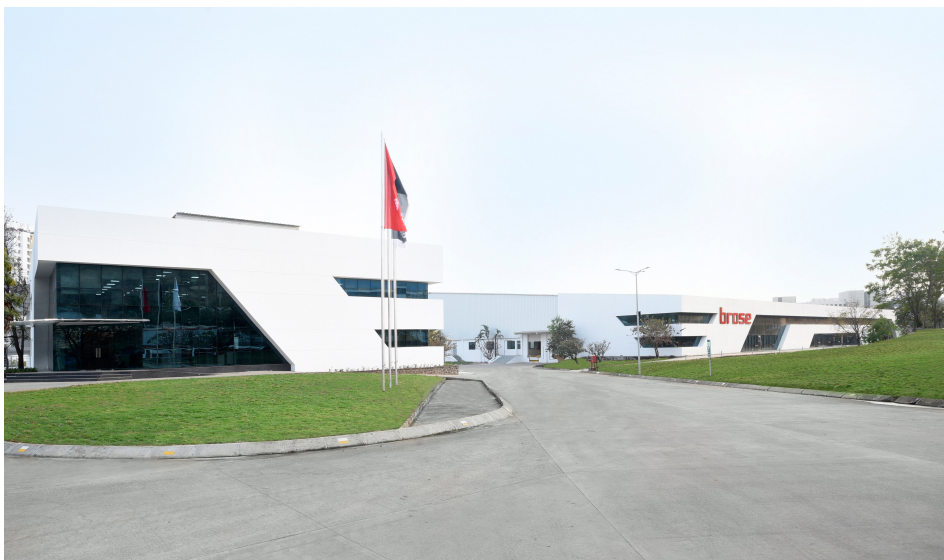
480 employees working at the new Brose location in Pune in development, production and administration.
